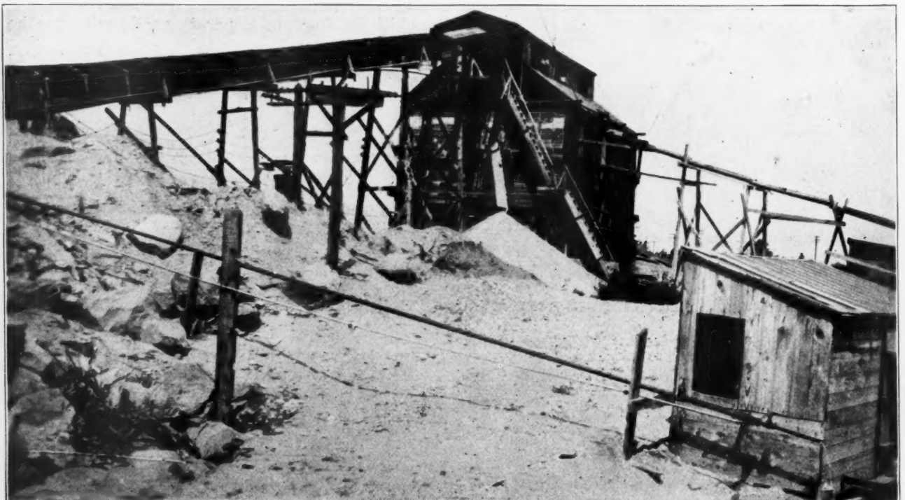
Conveyor to Sizing Screens with Pump House at Right
